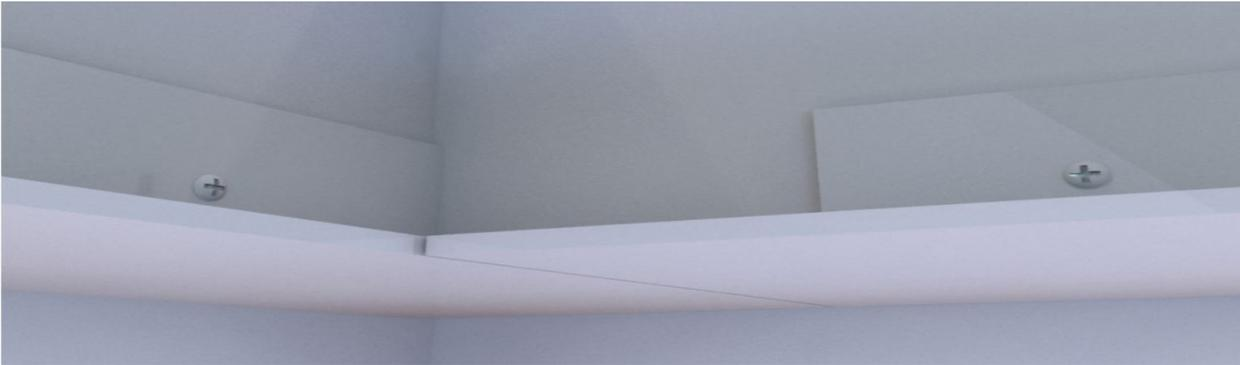
7. Remove 3 of the Angle profiles leaving the angle in place which is at the head of the blind
