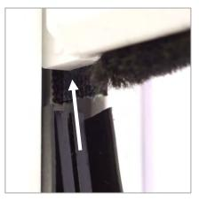
Engage the zip at the bottom of the hembar, with the opening at the centre of the plastic insert.
