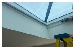
3. Prop the blind clear at both ends to make room to fix the end L-profiles
