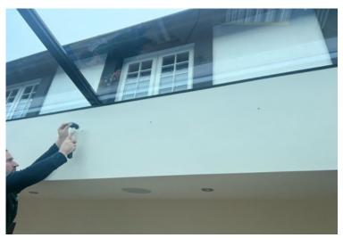
3. Drill and plug with a 6.5mm drill bit and plugs.
