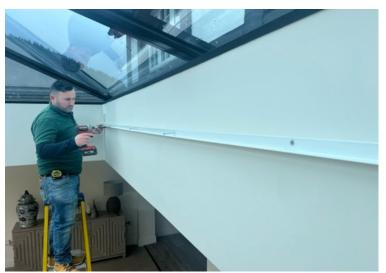
4. Affix both side L-profiles to the wall. The top and bottom rails will be fixed after the blind is in position.
