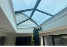
Lift the blind and tilt to clear the side L-profile as illustrated.
