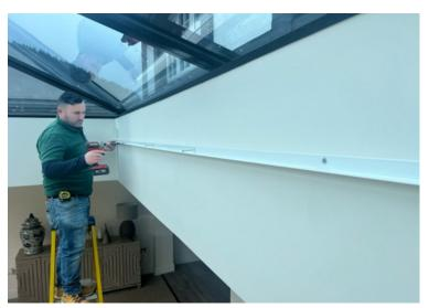
Affix both side L-profiles to the wall. The top and bottom rails will be fixed after the blind is in position.
