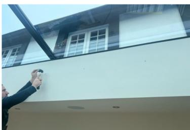
3. Drill and plug with a 6.5mm drill bit and plugs.
